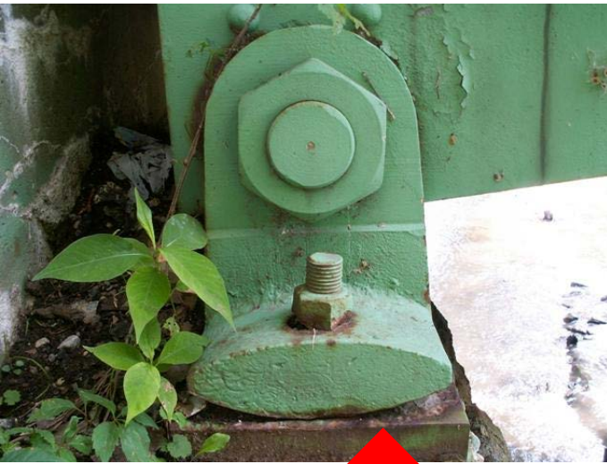
Pinned Rocker Bearing
