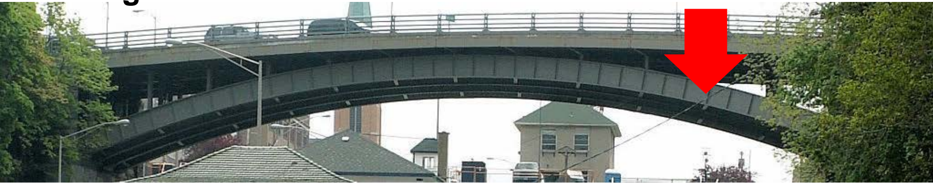
Deck Arch With Solid Rib
