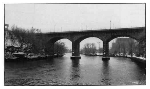
but the sides of the bridge are built of irregularly shaped stone. The arches themselves are constructed of brick. Cushing & Company of Providence designed the bridge and Pawtucket mason Horace Foster built it. Its impressive size, fine stone work, and original ironwork make Division Street Bridge a significant example of nineteenthcentury masonry arch construction.
