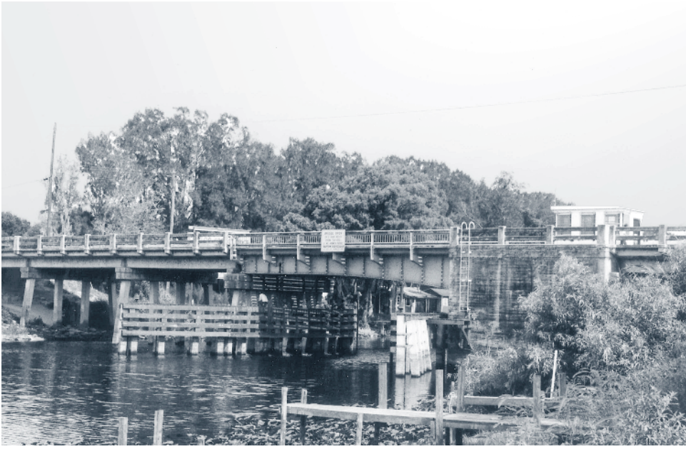
The Taylor Creek Bridge in Okeechobee County is a trunnion type bascule bridge.
