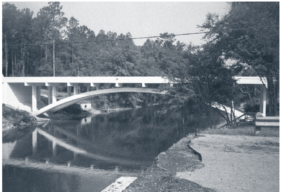
The Willis Bridge in Calhoun County is the only open spandrel arch in Florida that serves as a highway bridge.
