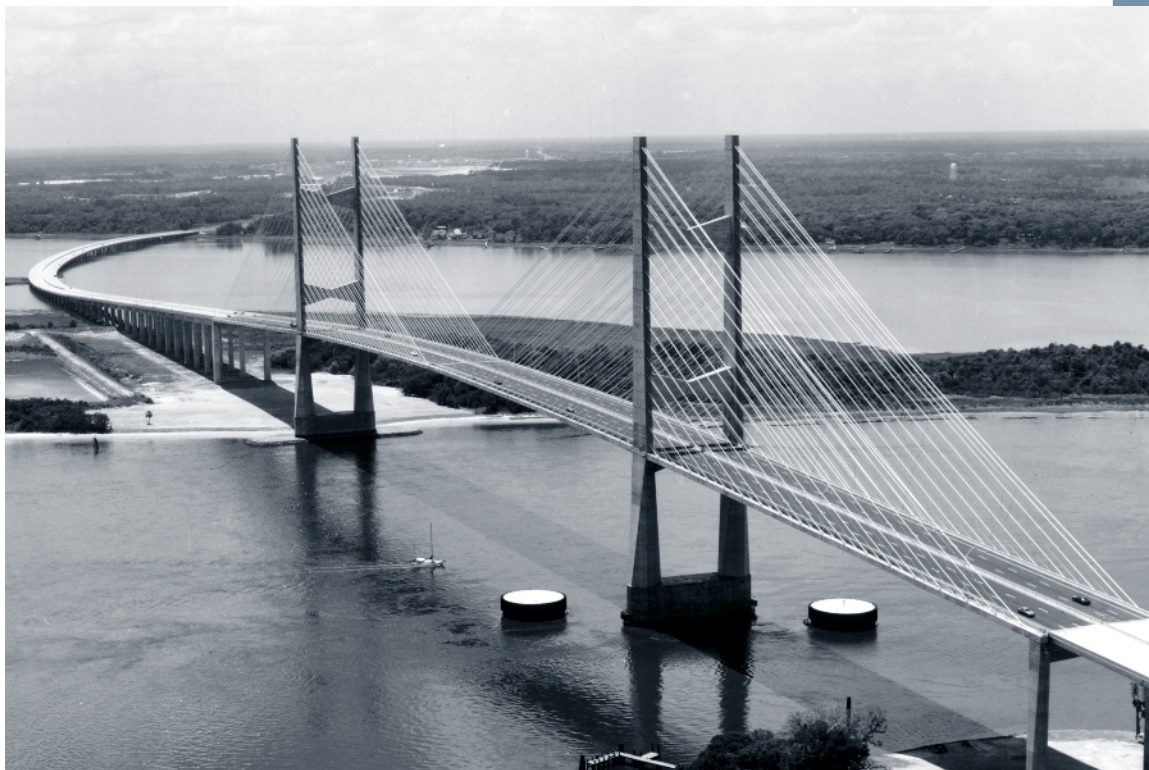
The Napoleon Bonaparte Bridge at Dames Point on the St. Johns River near Jacksonville features a harp stay arrangement.
