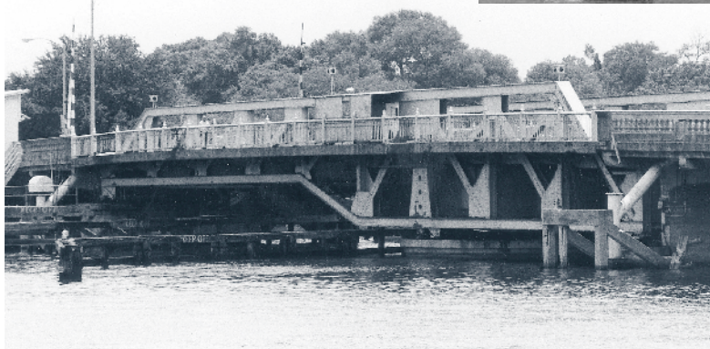
The Mt. Vernon Bridge Company of Ohio, an important Florida bridge builder, fabricated and installed the Michigan Avenue Swing Bridge across the Hillsborough River in Tampa in 1926. It sports an unusual bob-tail swing main span with a distinctive Warren pony truss.
