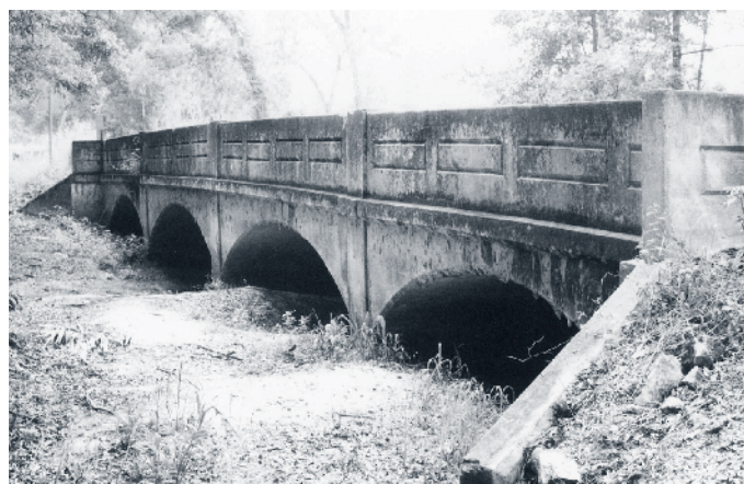
In the early 1920s, probably 1920 or 1921, Volusia County contracted with the Luten Bridge Company to build this four-span, reinforced concrete arch deck bridge on Deep Creek . The bridge once occupied a key location on a locally important roadway, called the St. Johns River Scenic Road.
