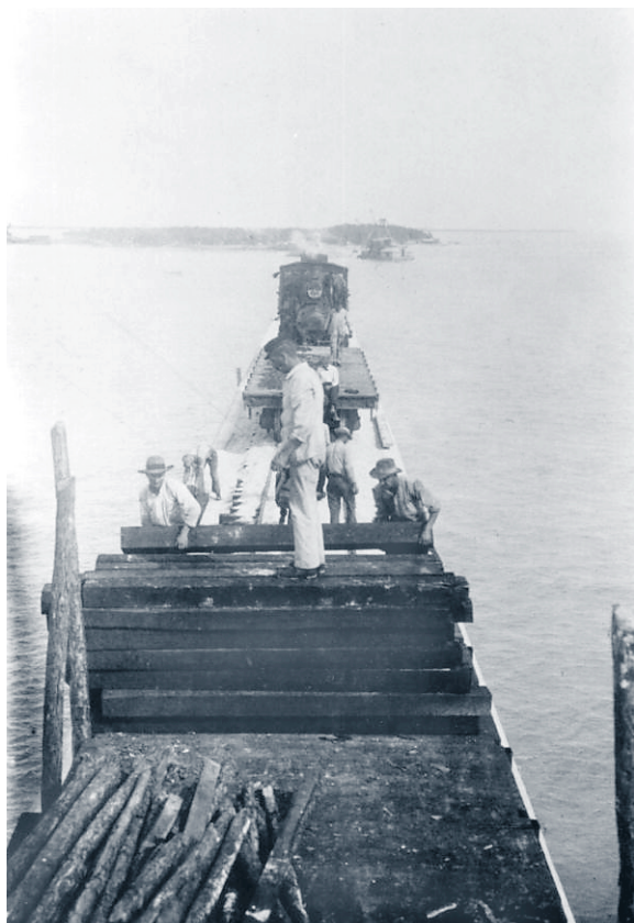
Railroad construction crew distribute cross ties on the Long Key Viaduct, 1907
