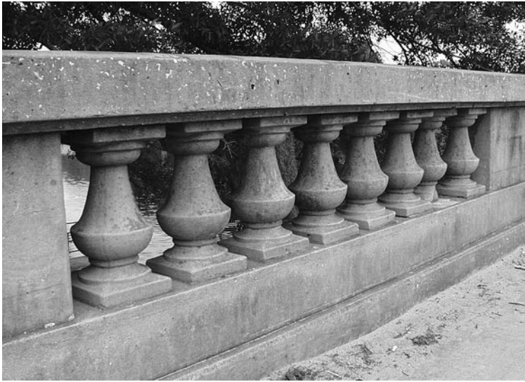
Detail of cast concrete balusters on the James N. Holmes Bridge in Hillsborough County
