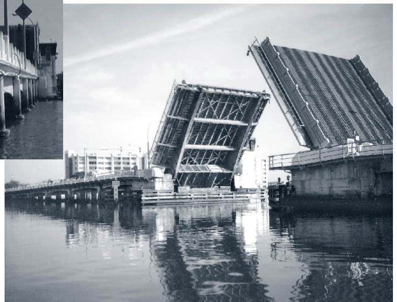
Another view of the Treasure Island Causeway showing open bascule
