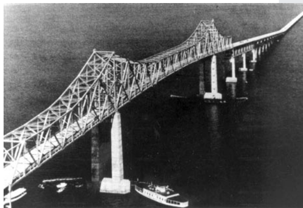
Photo showing the original Skyway Bridge that was damaged and consequently replaced when a freighter caused the collapse of its center span.
