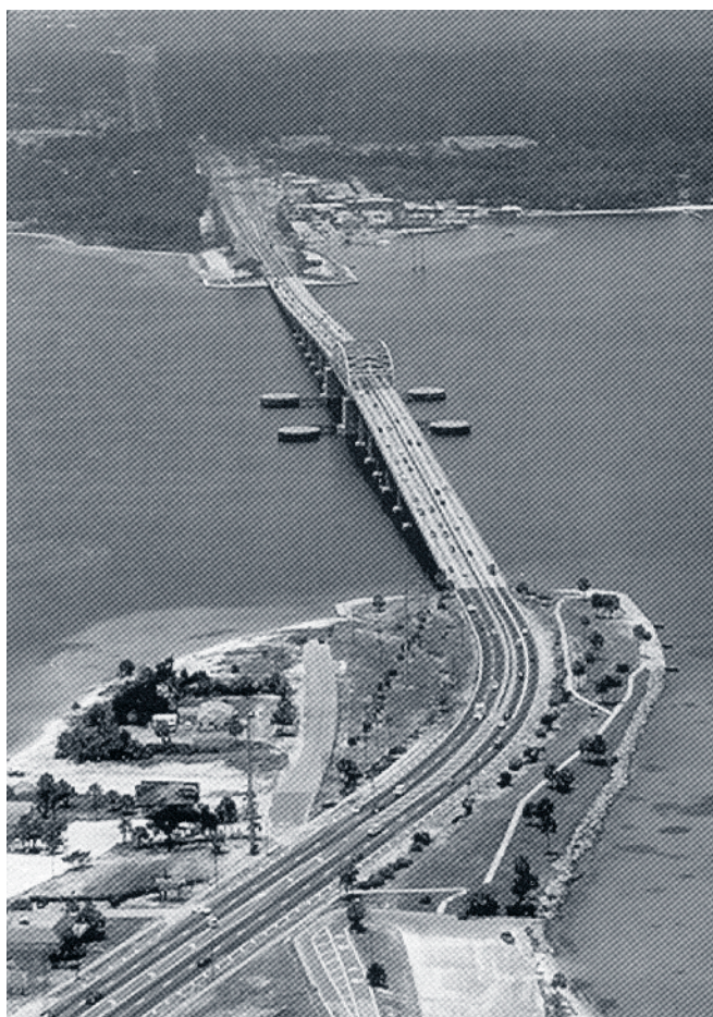
The Hathaway Bridge in Panama City features the largest number of single-cell boxed segments in the U.S.
