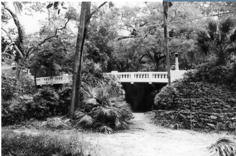
The Washington Street Bridge, a fine example of a reinforced concrete arch deck bridge
