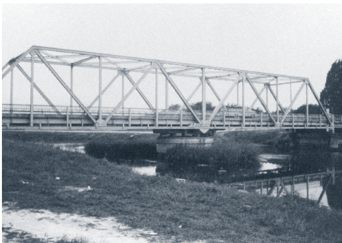
The Twenty Mile Bend Bridge, or Loxahatchee River Bridge (above), features a 188-foot-long Warren through truss mounted on a center-bearing pivot. The steel for this bridge carries the mill marks of "Carnegie U.S.A."
