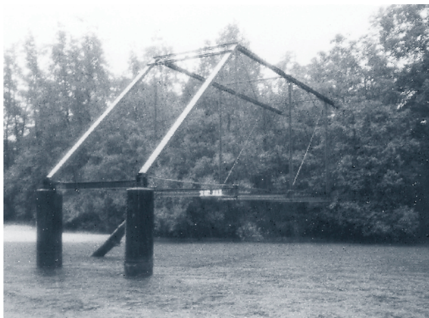
The Coldwater Truss is a fixed through truss located just outside of the Blackwater State Forest, just off State Road 191. Little remains of this abandoned structure and no evidence of the former associated road exists. It is one of only four Pratt-type through trusses remaining in the state and appears to date from the first two decades of the 20th century.
