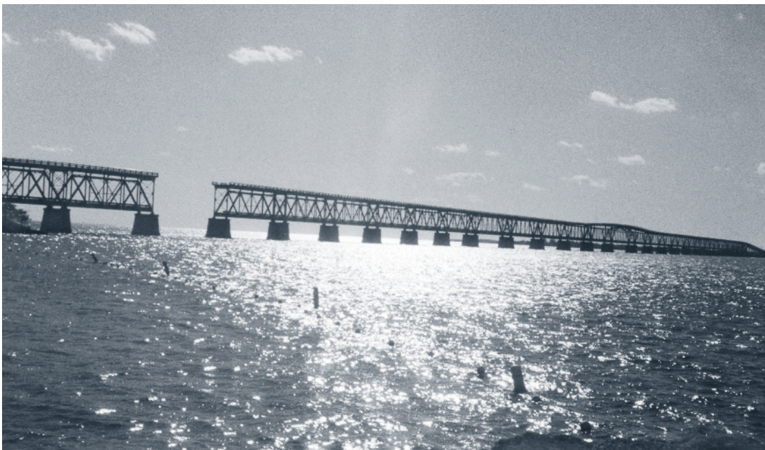
Bahia Honda Bridge with section removed to accommodate water traffic
