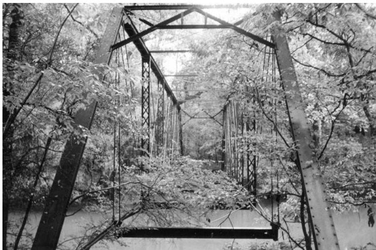
The 1914 Bellamy Bridge over the Chipola River, north of Marianna, derives its name from a nearby plantation. This Converse Bridge Company structure was shipped in parts by rail and quickly and inexpensively erected on the site.
