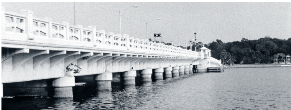
The Ortega River Bridge reflects the trademark Maltese cross design and decorative tender stations of bridge engineer T. B. Carrick.
