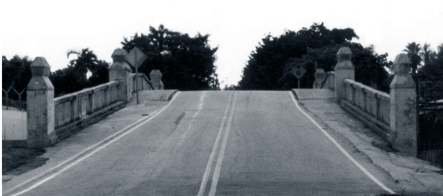
Associated with the development of Spring Garden, the Seybold Canal Bridge represents an interesting example of an early concrete arched design. This barrel arched bridge has a pronounced arched rib, and large, geometrically-shaped, concrete caps top the heavy, square abutments.
