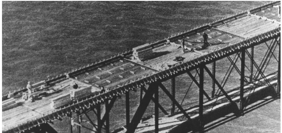
Historic photo showing the conversion of the Bahia Honda Bridge from a railroad into a highway
