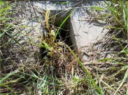
A photograph of a shoulder drain opening. The drain is blocked by a large pile of dry, brown vegetation and debris, with some water pooling around the opening.                                                            | A18                |
