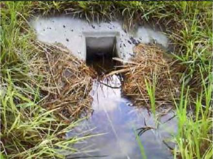
A photograph showing a shoulder drain opening. The drain is heavily obstructed by dry vegetation. There is significant erosion around the drain, with a deep, narrow channel of water flowing through the debris and soil. | A17                |
