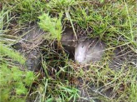
A photograph of a shoulder drain opening surrounded by tall green grass. The drain is almost completely blocked by a thick layer of dry, tangled vegetation and debris.                                                     | A16                |
