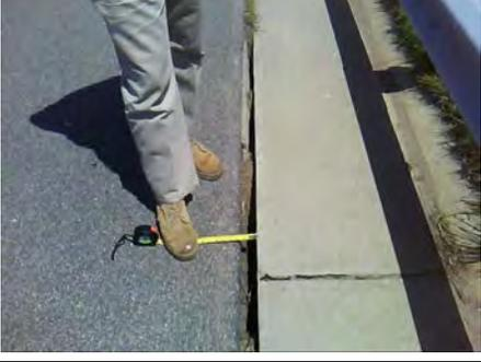
A photograph showing a person's legs and feet standing on a road surface. A yellow measuring tape is held against the edge of a concrete curb, showing a clear gap between the curb and the road pavement.                     | A37                |
