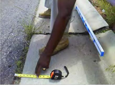
A close-up photograph of a person's hand using a yellow measuring tape to measure the gap between a concrete curb and the asphalt road surface. A blue level is also visible, indicating the curb is not aligned with the road. | A4                 |
