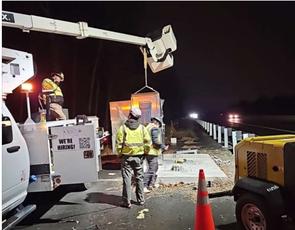
➤ Installing the toll equipment cabinet at AET 2.1 (A03)
