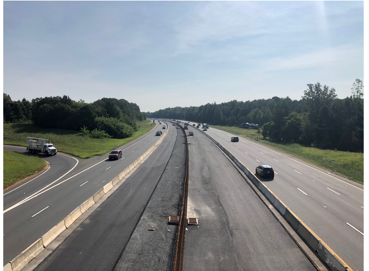
Segment C Median Widening near Providence Road
