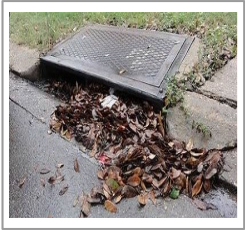
Clogged Catch Basins & Pipes 253
