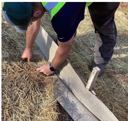
Image of WattleFence™ being installed in Rutherford County (left) and an image of a completed installation (above) from Western Excelsior's product data sheet.
