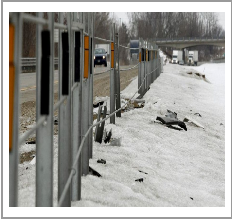
Bent/Torn Cable Rail
