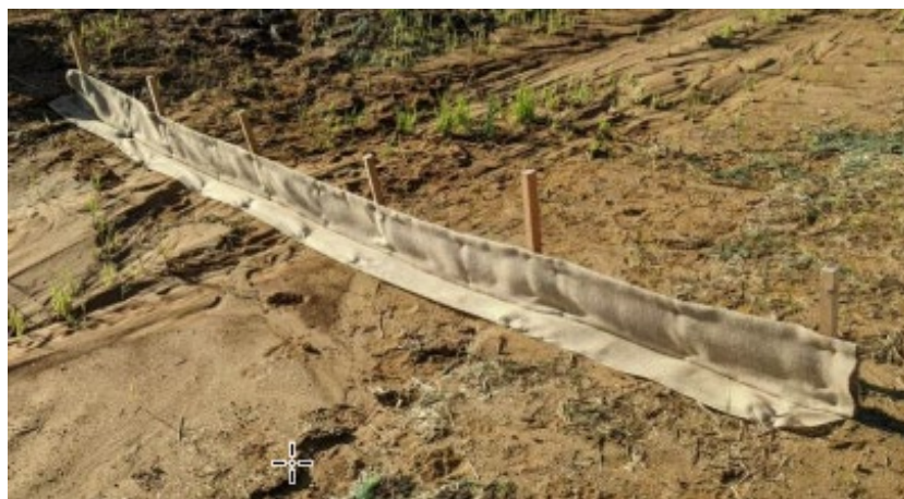
Image of WattleFence™ being installed in Rutherford County (left) and an image of a completed installation (above) from Western Excelsior's product data sheet.
