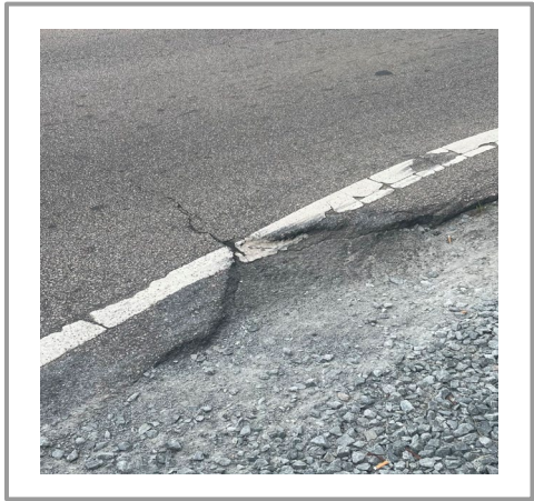
Collapsed Shoulder
