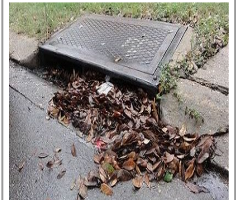
Clogged Catch Basins & Pipes
