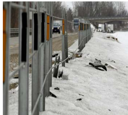
Bent/Torn Cable Rail
