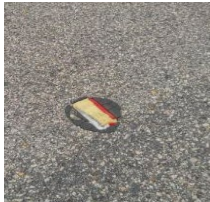
Missing Pavement Marker
