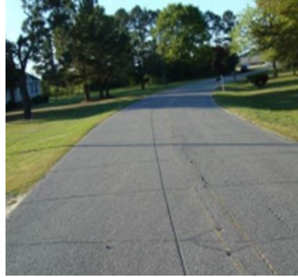
Faded/Missing Striping
