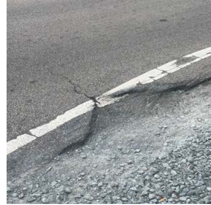
Collapsed Shoulder
