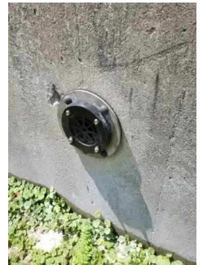
Images of the three models of Jet Filter Systems [left] and a Jet Filter System installed in a concrete structure [bottom] from Jet Filter System's website.
