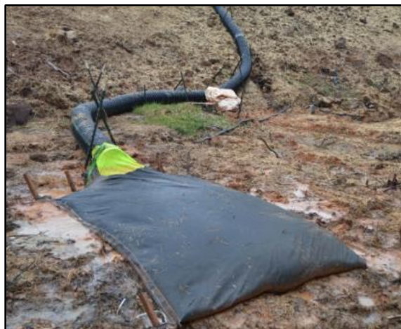
Slope Drain Bag installation on a jobsite – image from Silt-Saver® website
