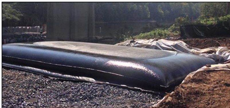
Example of a DirtBag®55 Dewatering Bag being used on a construction site – image from ACF Environmental website
