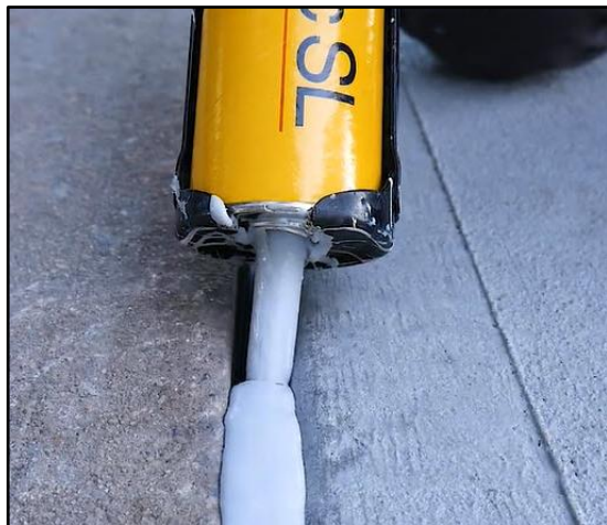
Sikaflex®-1A being used to seal the joint between an existing and a freshly poured concrete slab – image from Sika website
