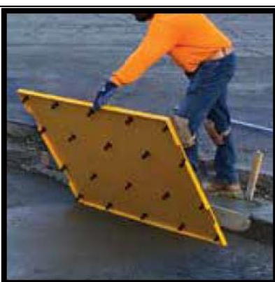
Side view of the AlertCast® CIP PAVER showing the perimeter flange (left), a worker installing the AlertCast® CIP PAVER with its black PENETRATOR® anchors protruding into fresh concrete (right) – images from DWS website
