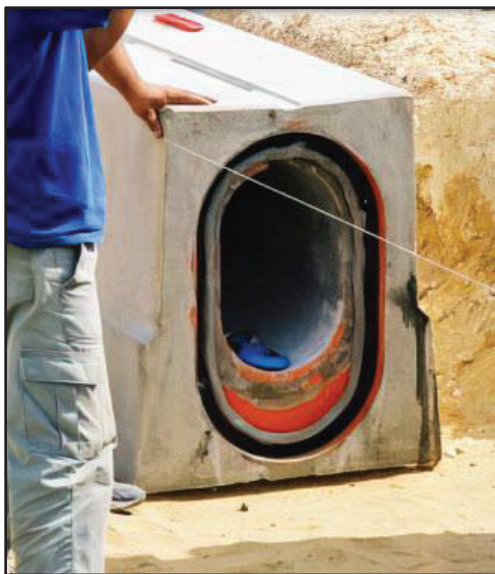
Installation of CS-440 on concrete pipe joints during installation of a stormwater drainage system at Ben Gurion International Airport in Tel Aviv, Israel – image from ConSeal™ website
