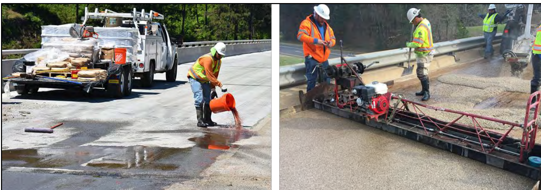
Worker pouring and rolling primer resin on the bridge deck (left), Workers pouring and leveling PCC 1121 on a bridge deck after the primer is applied (right) – images from Kwik Bond Polymers website
