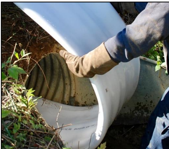
Worker pulling the Warrior Thermoform pip-liner through a metal pipe – image from Thermoform Website
