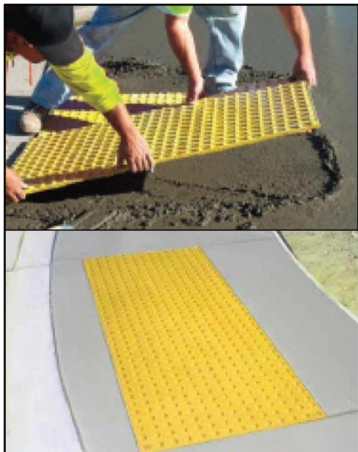
Workers placing an Equal Tile Paver in freshly poured concrete (top), an Equal Tile Paver in finished concrete (bottom) – images from Equal Tile brochure
