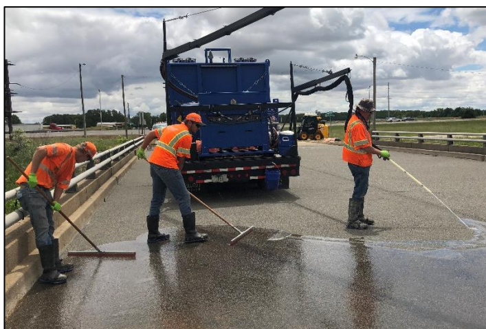
Workers applying and spreading E-TUFF® 7097 on a bridge deck – image from PSI
