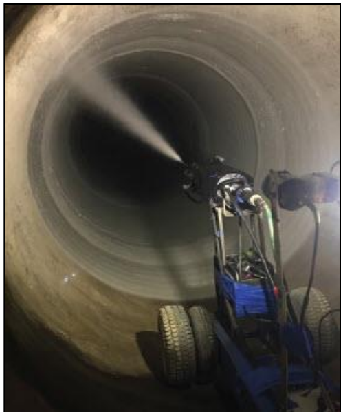
Application of Spray-Applied Pipe Liner using the 360Ringtech® Robot – image from 360Ringtech® brochure
