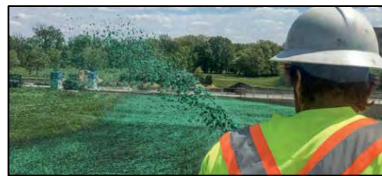
Application of Profile® HP Hydraulic Mulch products – image from Profile® HP Mulch brochure
