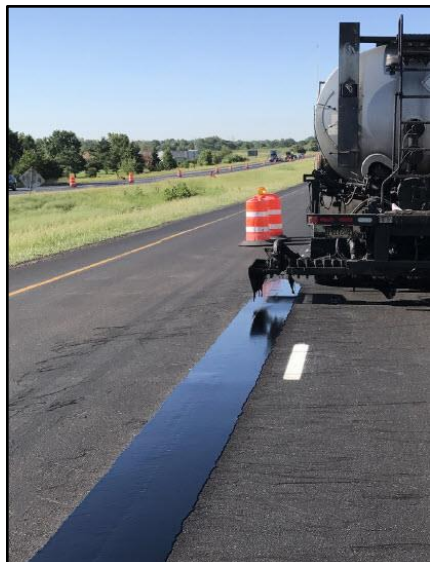
J-Band Longitudinal Joint Sealer being applied – image from Asphalt Materials, Inc. brochure
