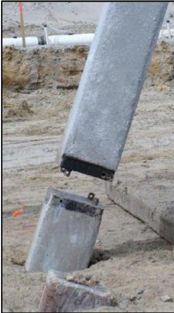
Two concrete piles with an EMECA Splice on each end about to be joined in the field - image from EMECA/SPE USA Brochure
