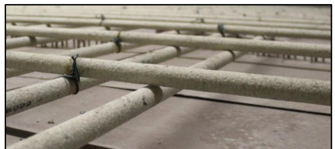
Grey/white BFRP rebar tied together prior to a concrete pour for a parking garage floor – image from Pultrall twitter account
