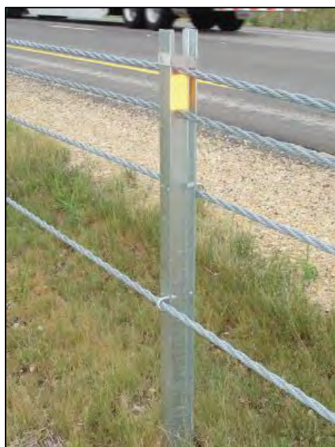
CASS® S3 M10 TL-3 and TL-4 median cable barrier system installed along a highway median - image from Trinity website
