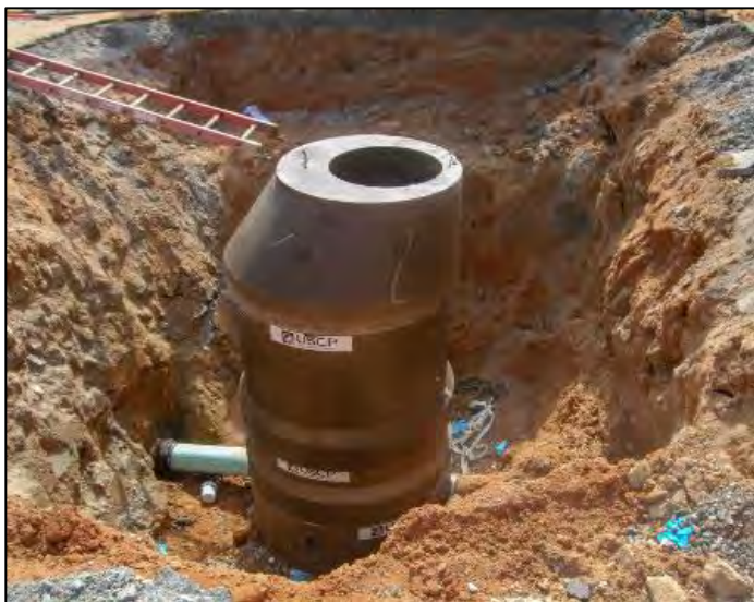
Installation of USCP Steel Reinforced Polymer Manhole – photograph from USCP website
