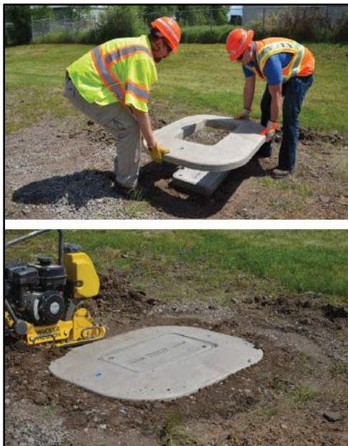
Installation of a Quazite® Box Collar around a utility box by two individuals (top photo), finished installation after backfilling and soil compaction (bottom photo) – images from Quazite Brochure
