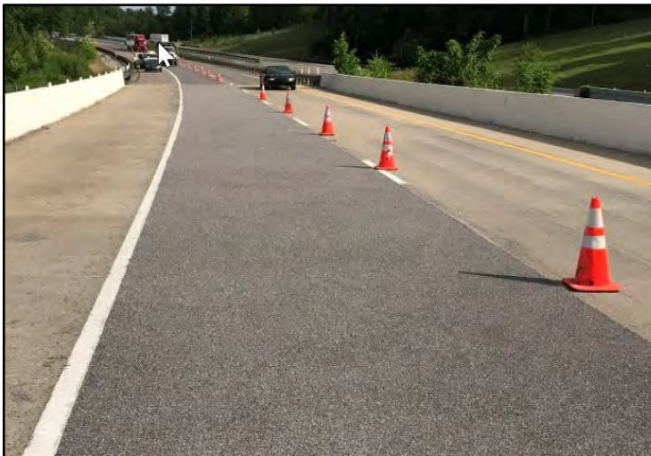
View of HFST aggregate overlay using SAFE-T-GRIP® 1:1 epoxy polymer on a concrete bridge deck – photograph from EPOPLEX website
