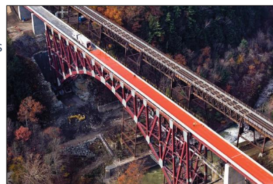
Aerial view of BDM being applied to a new railway bridge – image from BDM brochure
