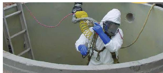
Installation of SprayWall® in a vertical concrete pipe – image from SprayROQ™ website
