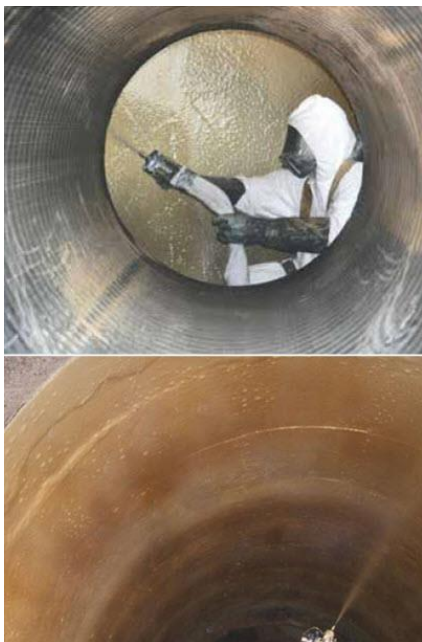
Installation of SprayWall® on steel pipe (Top), Installation of SprayWall® on concrete pipe (Bottom) – images from SprayROQ™ website
