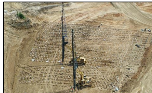
Installation of PVDs by two specialty equipped excavators – image from Geoengineer.org website
