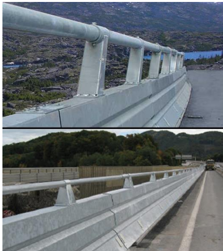
TL5 Barrier installed (Top), TL4 Barrier installed (Bottom) – image from MDS® Brochure
