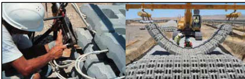
Worker connecting concrete blocks together to form ArmorFlex® mat (left image), machine placing mats of concrete blocks into place with equipment (right image) – images from ArmorFlex® brochure
