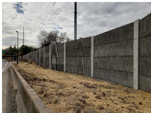
Example of standard AcoustaCrete – image from Faddis website
