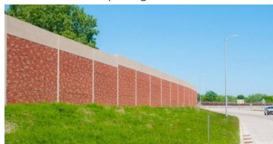
Example of brick textured AcoustaCrete – image from Faddis website
