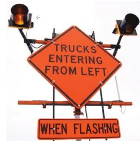
*Solar Advanced Warning Ingress/Egress System with construction truck warning sign – image from SAWS*
