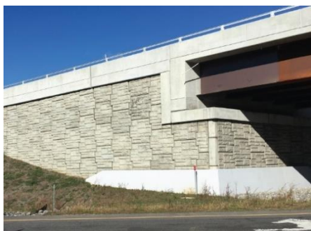
Example of MSE Wall at a bridge approach – image from Google image search
