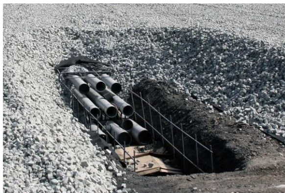
FGA G15 placed over underground utilities – image from Aero Aggregates' website
