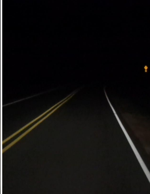
4" Standard Bead Thermo SR 1116 (Cedar Creek) Franklin Co. Installed 2012 (Estimated) Photo Taken Dec 2017 (Retro Data: CL 181/EL 336)
