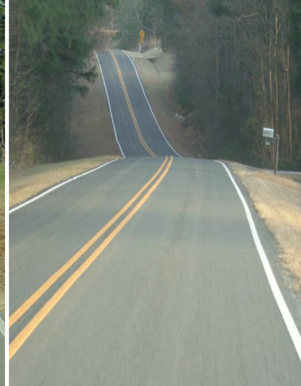
NEW 4" Standard Bead Thermo SR 1131 (Tump Wilkins) Granville Co. Installed Summer 2016 Photo Taken Dec 2016 (Retro Data: CL 308/EL 470)
