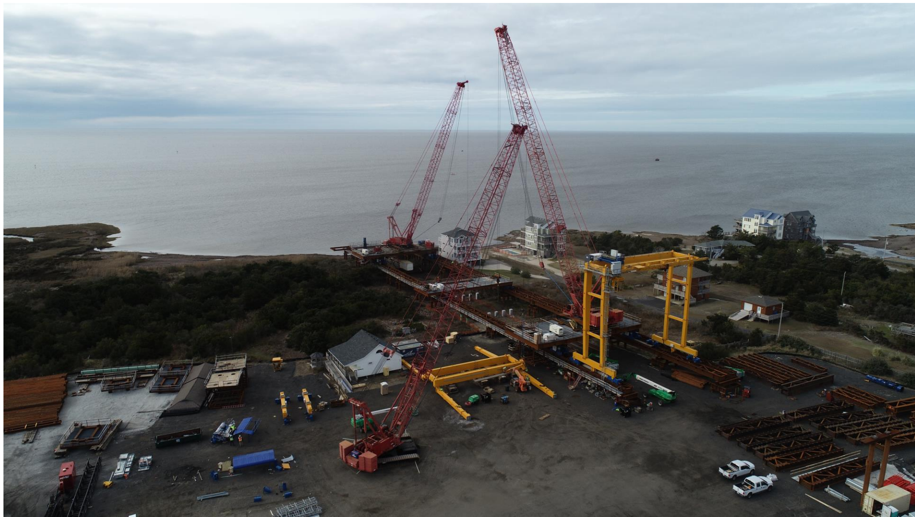
Assembly of Rail and Gantry System at South End
