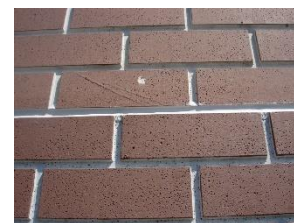
Durisol's Noise Barrier cast in a brick pattern
