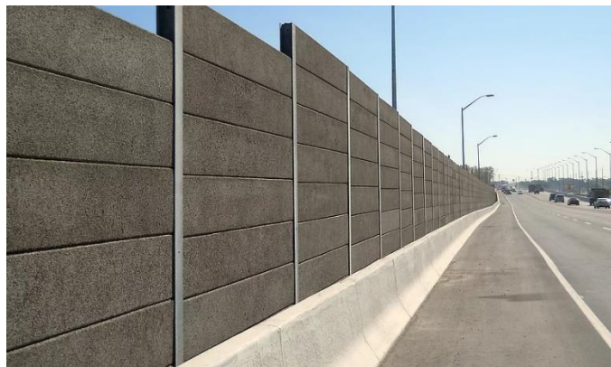
Image of Durisol's Precast Noise Barrier from their website
