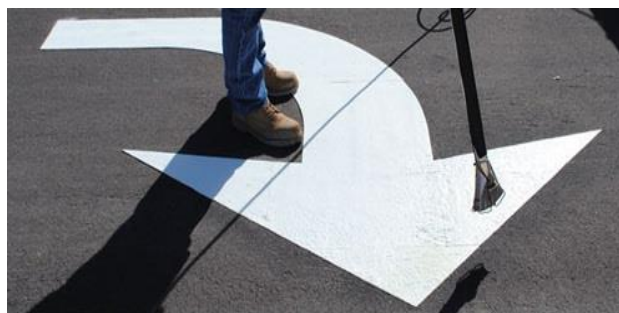
Preformed thermoplastic arrow bonded to pavement using a torch – image from Google
