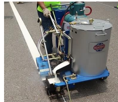
Thermoplastic markings being applied by cart – image from Google
