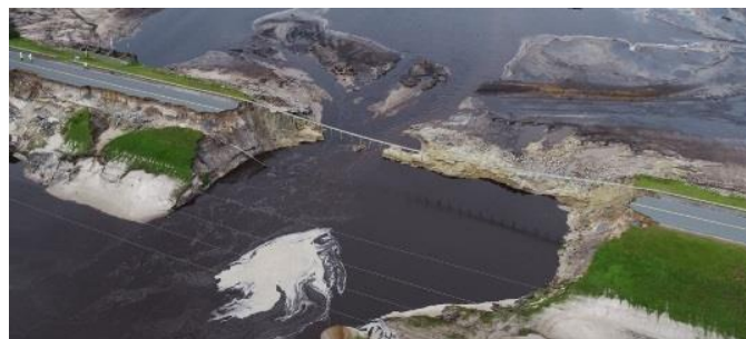
Drone footage of dam breach at Boiling Springs Lake, NC
