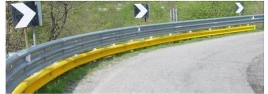
*DR-46 Motorcycle Barrier Attenuator installed on a roadway curve.*
