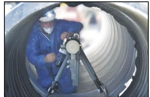
Centri-Cast Pipe Repair Mortar being applied.
