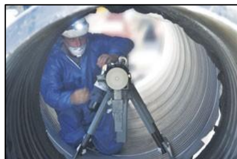
Centri-Cast Pipe Repair Mortar being applied.
