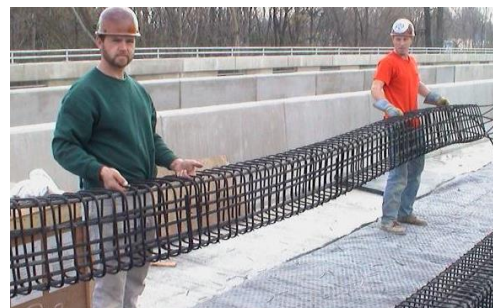
CFRP Reinforcement Cage
