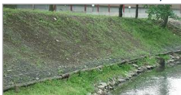
Ecoraster E50 Used for Slope Stabilization
