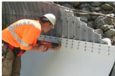
HCCR being installed on an existing culvert
