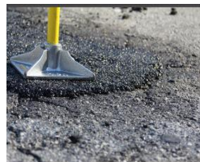
Example of QPR being compacted. From QPR
