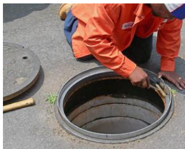
Example of installation of riser.
