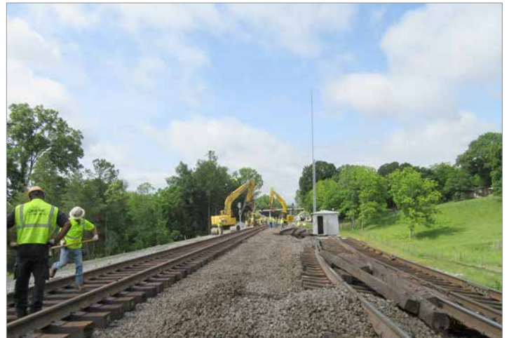
Removing CP Haydock from service and lining for second track
