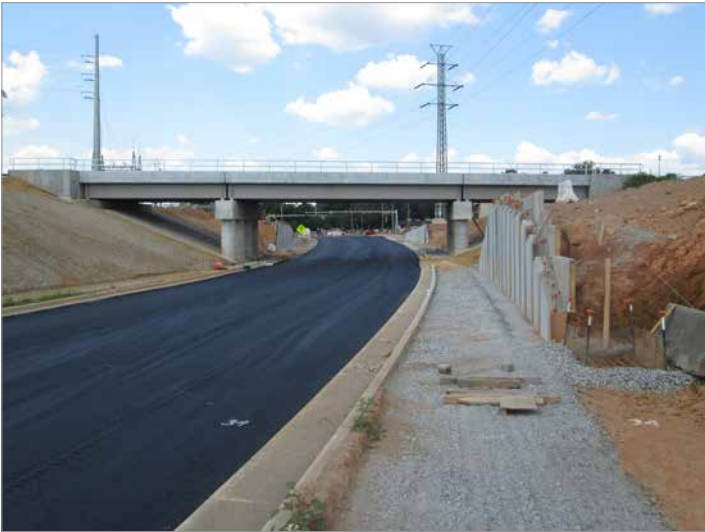
U-3459 Klumac Road, roadway paving
