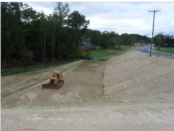
P-5204 McLeansville Road, final grading
