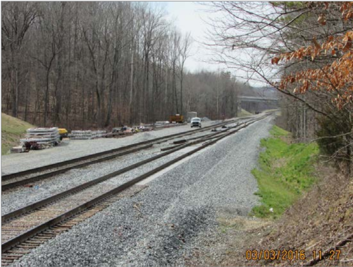
C-4901 Bowers to Lake, construction of second track
