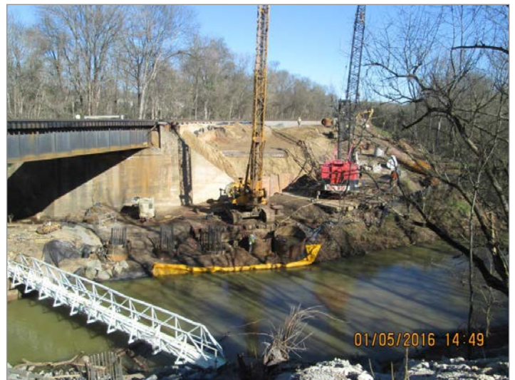
P-5208A Haydock to Junker, Coddle Creek Bridge, drilled shaft construction for north interior bent
