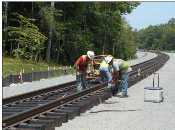
C-4901 Bowers to Lake, track Construction
