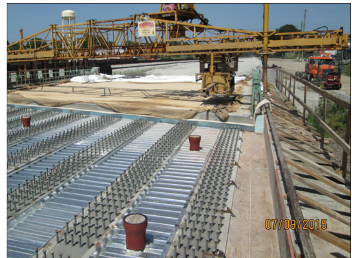
U-3459 Klumac Road, bridge construction
